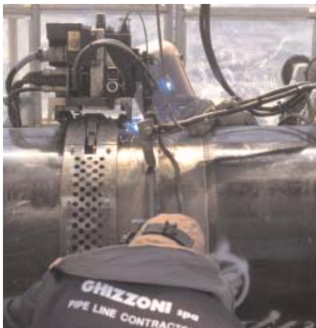
Figure 1. Mechanised pipe welding equipment running ESAB OK 12.65 EcoMig wire.
