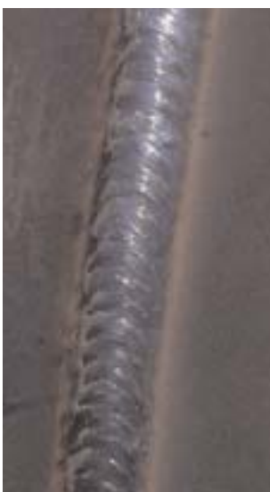
Figure 4. Finished weld. Filling and capping is done under 50%Ar/50%CO 2 mixed gas.
