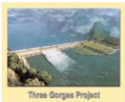
Figure 2. Overview of the Three Gorges dam project showing ship-locks (right), a spillway in the centre of the dam and power plants on the left and right banks (3).
