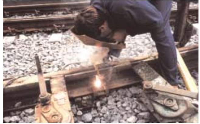
Figure 4. Welding of the rail foot.
